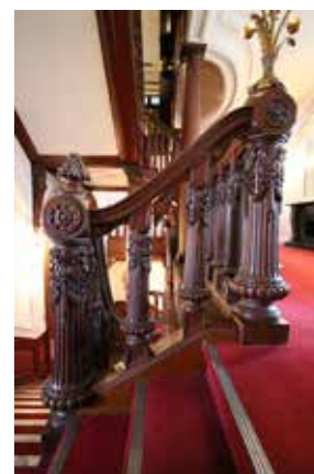
10-7 2階広間階段手摺
